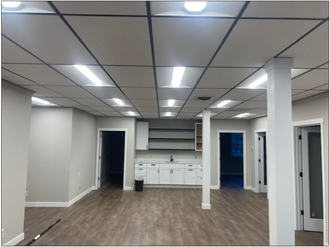
OLD CITY HALL INTERIOR
